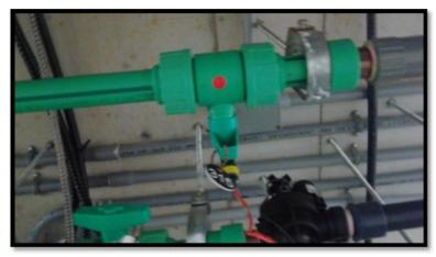
• Close valve #315 after approx. 20 minutes or just after water begins to run from the overflow pipe around the corner.
